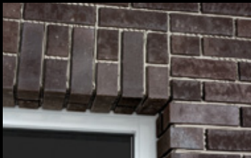
Window lintel perfectly replicated with angles.
